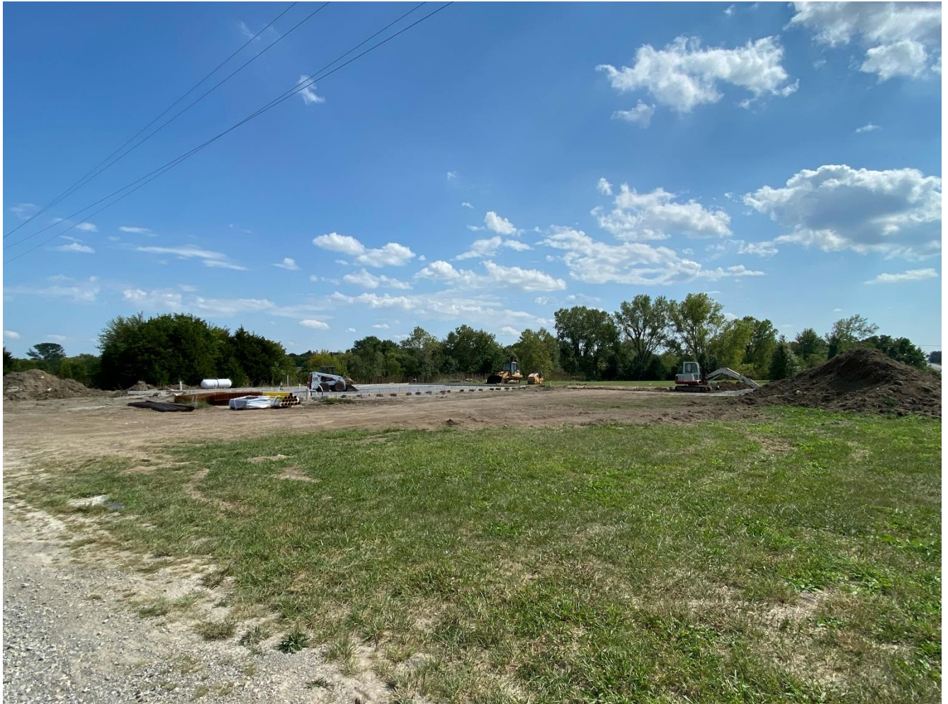
New Station 4 Construction – 9/17/2022
